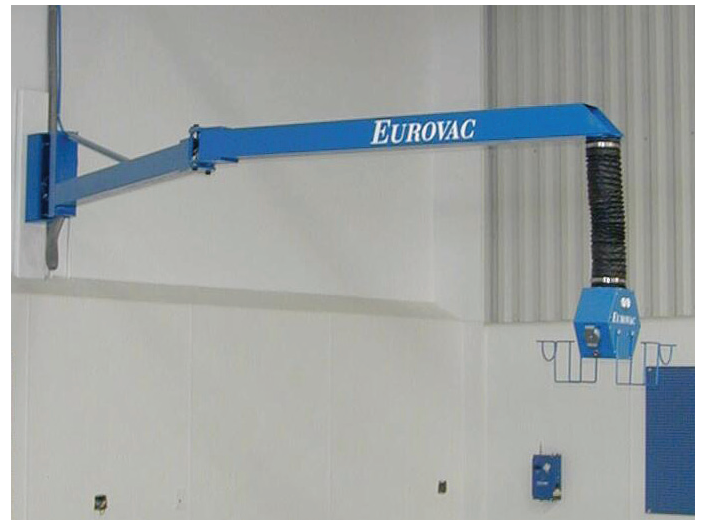
Articulated Booms & Pendant Drops with dual inlet, integrated compressed air and 110v electric
