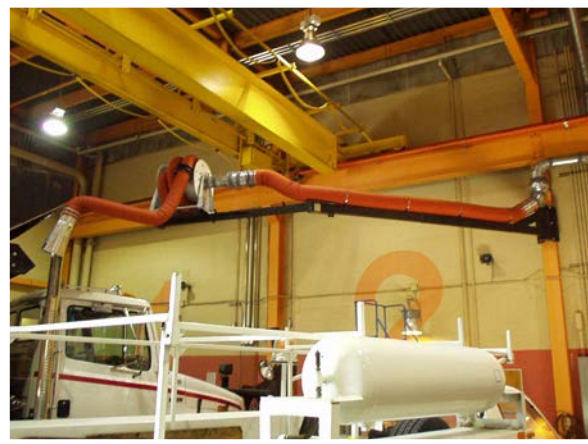
Extension pivot swing boom with hose reel for additional horizontal reach
