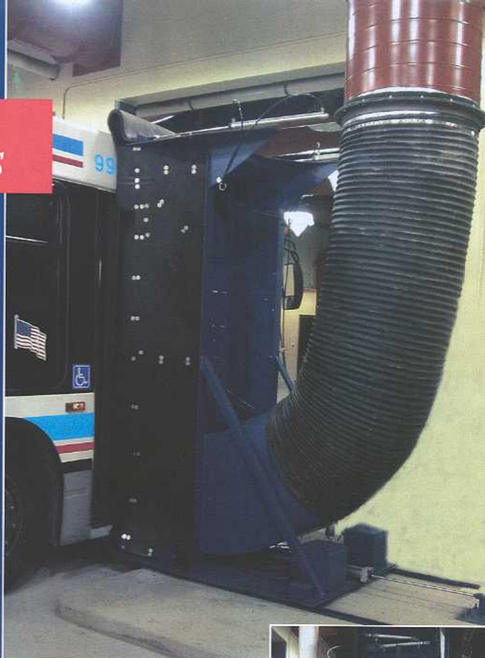
ABOVE: 30" Flex Hose attached to a retractable Bellows. RIGHT: Air Gun and Hose.
