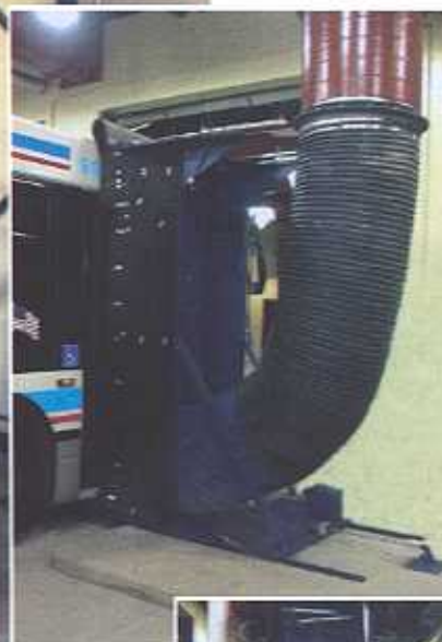
Retractable bellows (with air gun hose) extends and seals the bus door when the system is activated
